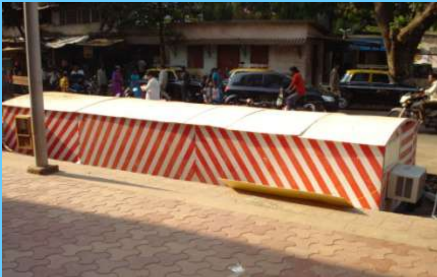
Cable Joint Chamber
