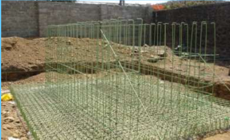
Traction Transformer Foundation Mahalaxmi
