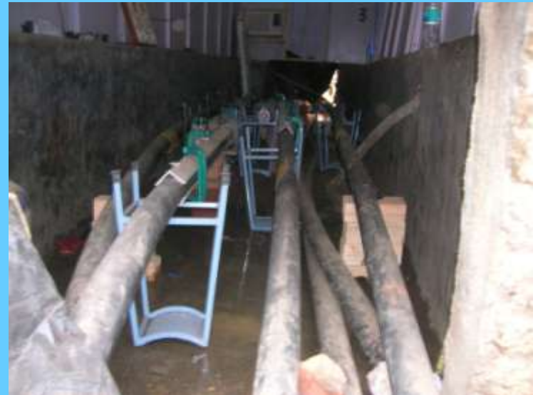
Inside view of Cable Joint Chamber
