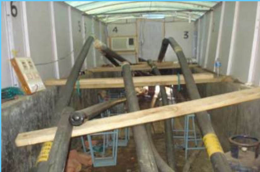
Inside view of Cable Joint Chamber
