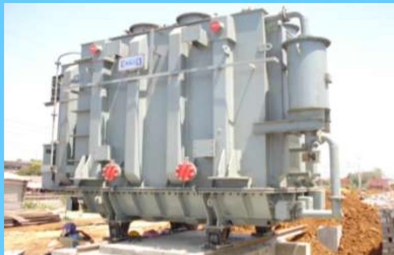
Traction Transformer Installation Jogeshwari
