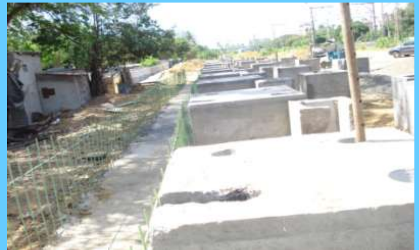
Goregaon - Equip Foundation & Cable trench
