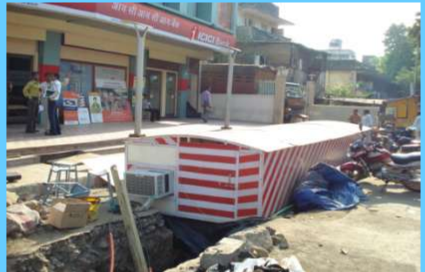
Cable Joint Chamber
