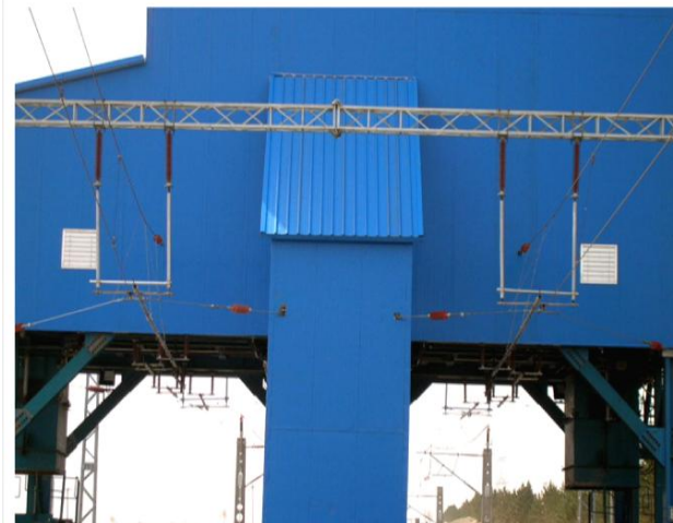
Figure 6: Load out in an electrified siding
